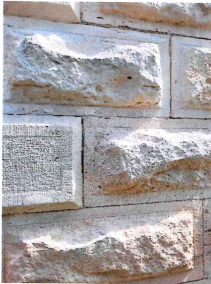
(Additional locations of missing mortar in joints)
