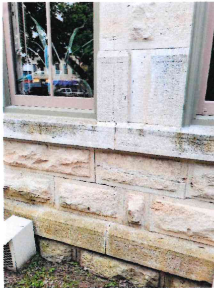
(Missing mortar joints throughout allowing water infiltration)
